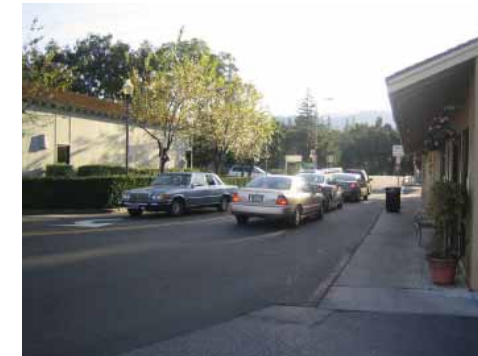
Heavy traffic, a flush sidewalk curb, and unclear definition of a right-turn lane creates an unsafe pedestrian condition at A Street.
