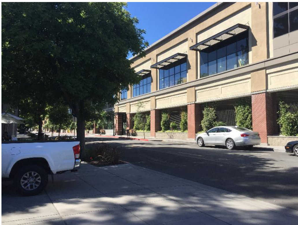
Photograph 6: View looking southwest toward 160 1 st along 1 st Street.
