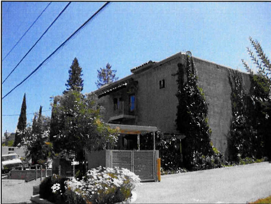
E09-581; rear view of property
