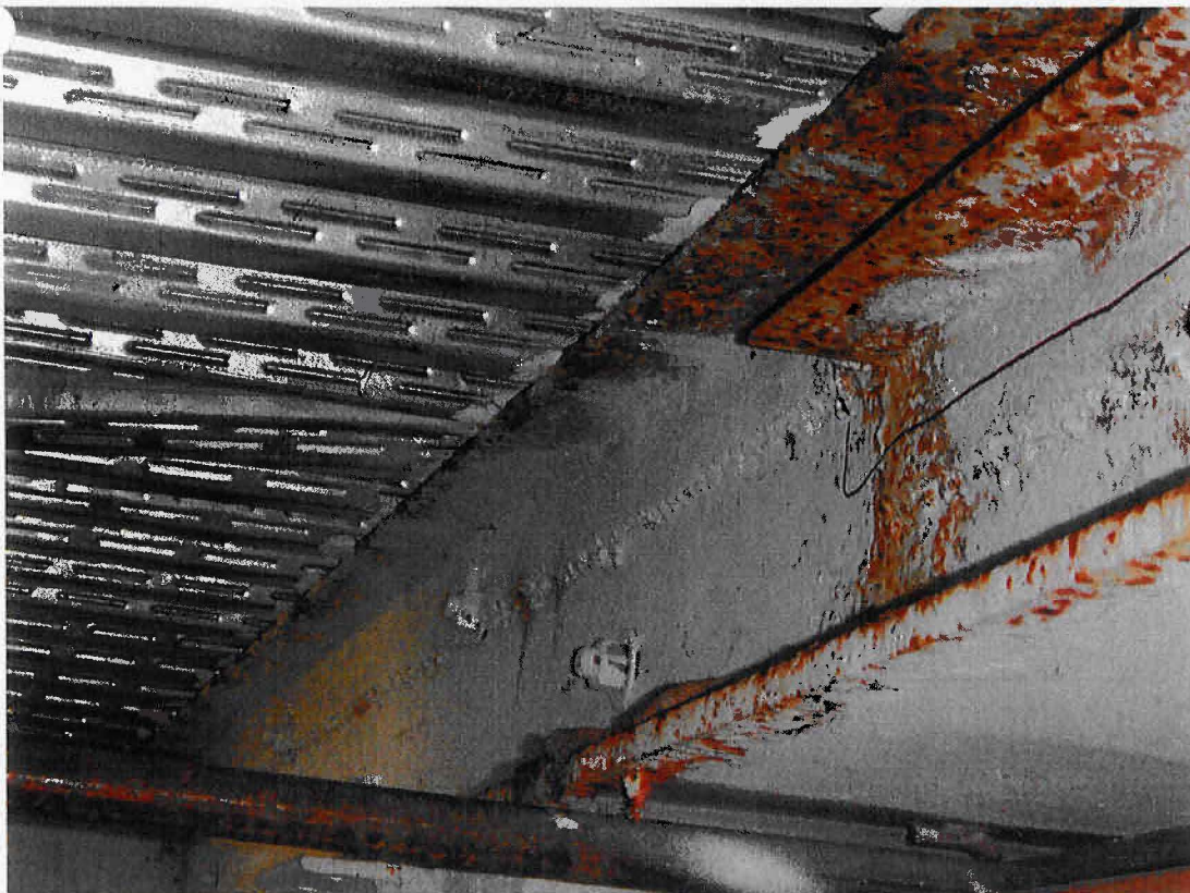
Basement Level - Small Storage Area
