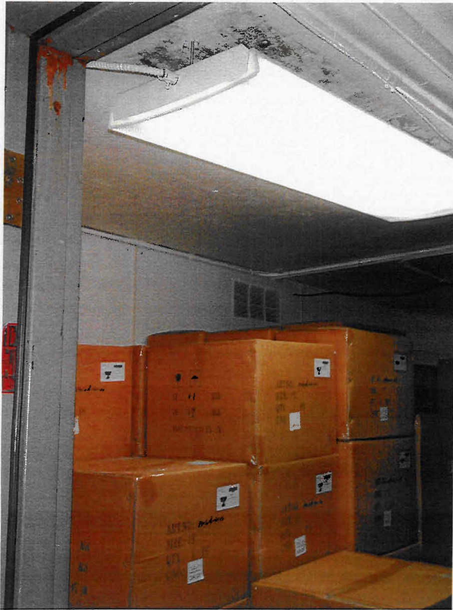
Basement Level - Dry Storage Area and Freezer Area
