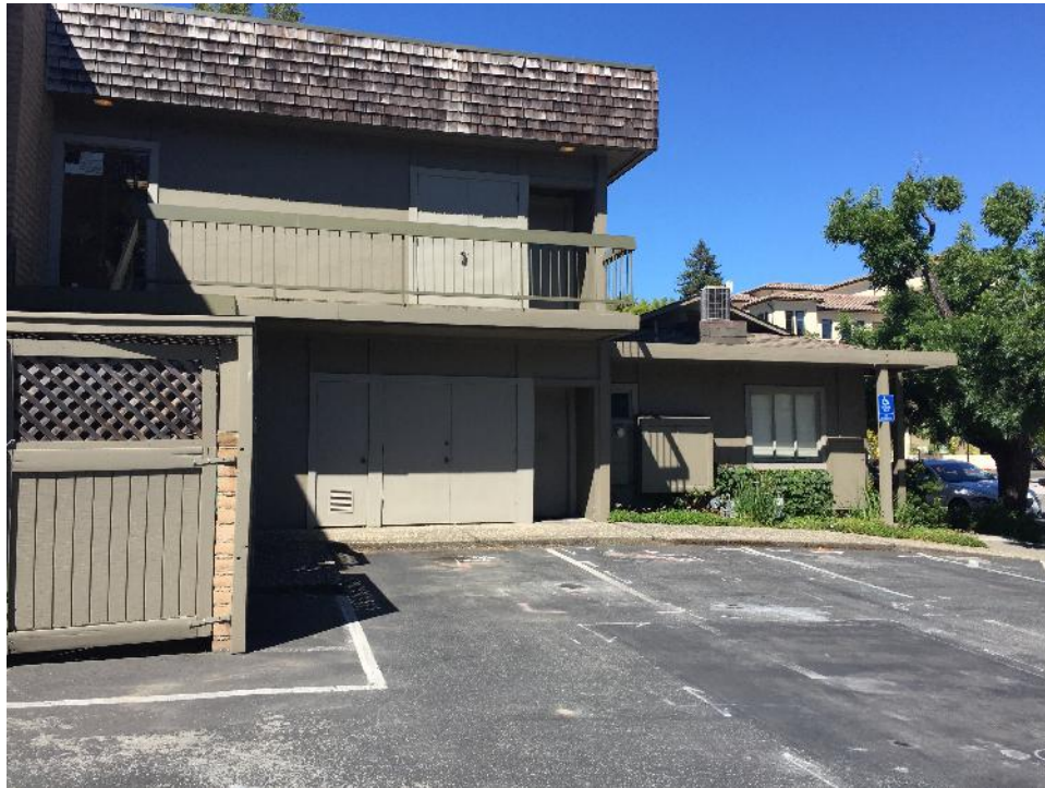
Photograph 1: View of rear of 101/111 1 st Street from alley.
