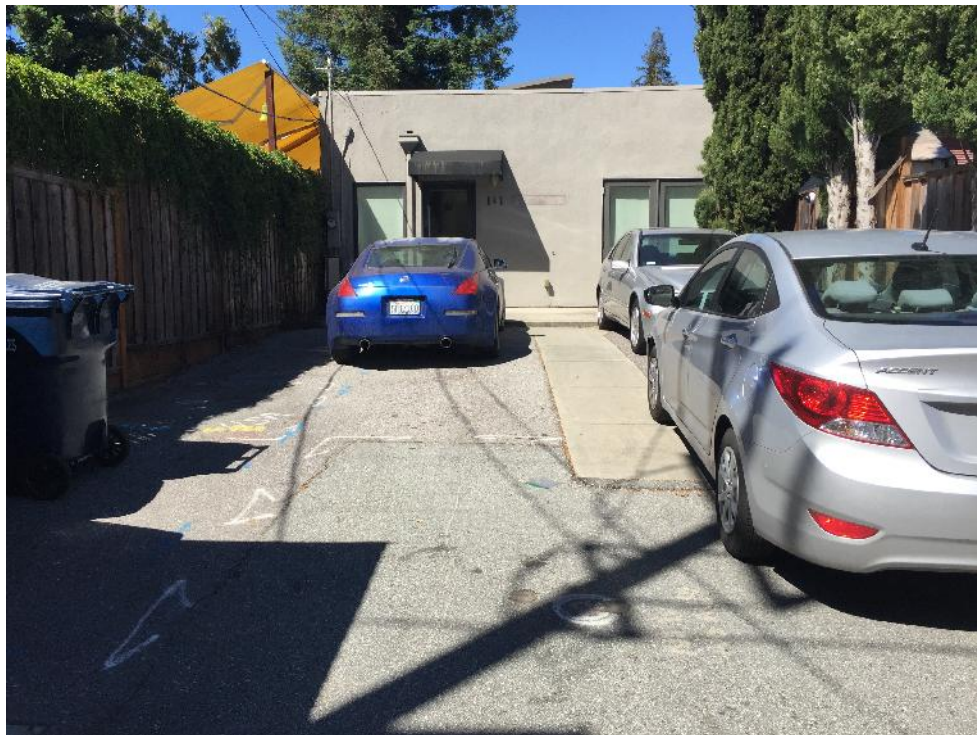
Photograph 12: View of rear of 141 1 st Street and former UST location.
