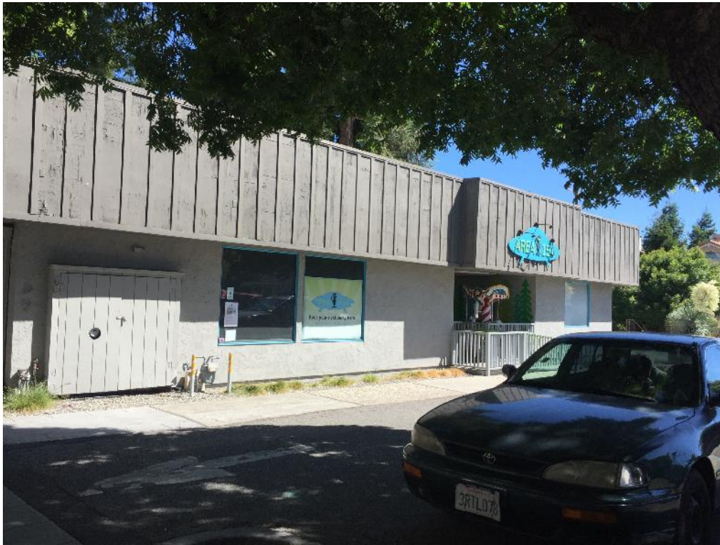
Photograph 13: View of 151 1 st Street from Plaza parking lot.
