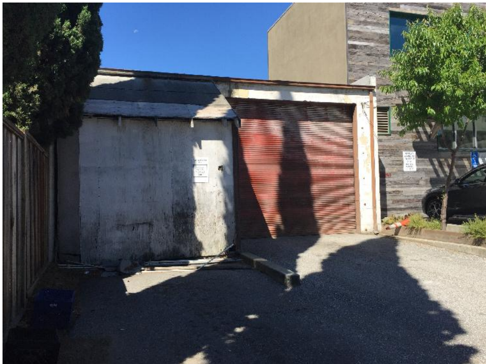
Photograph 10: Rear of 139 1 st Street.
