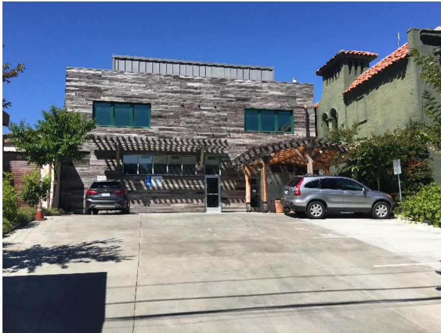
Photograph 7: View of the rear of 129 1 st Street.
