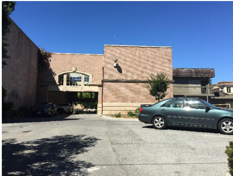
Photograph 4: View of the rear of 121 1 ST Street.
