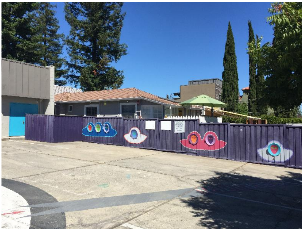
Photograph 14: View of rear of 151 1 st Street.
