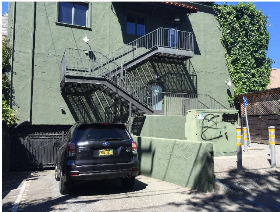
Photograph 6: View of the rear of 127 1 st Street.
