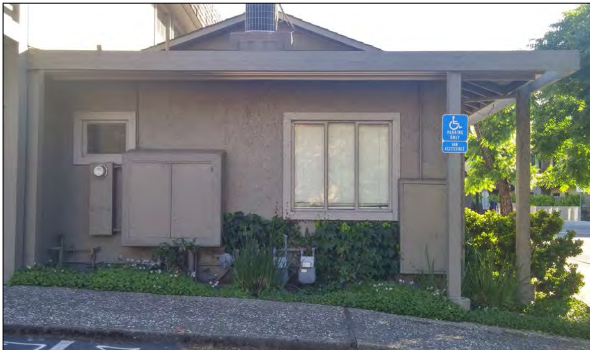
101 First Street, east façade. View to the west. LSA photograph 5/17/17.
