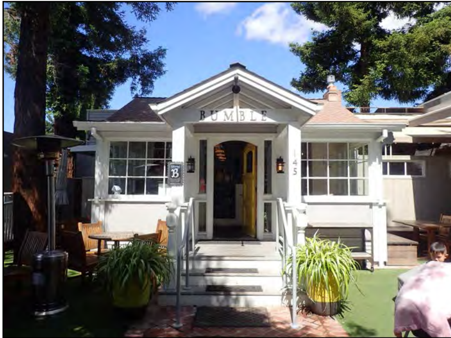
145 First Street, west façade. View to the east. LSA photograph 5/13/17. New covered entrance.
