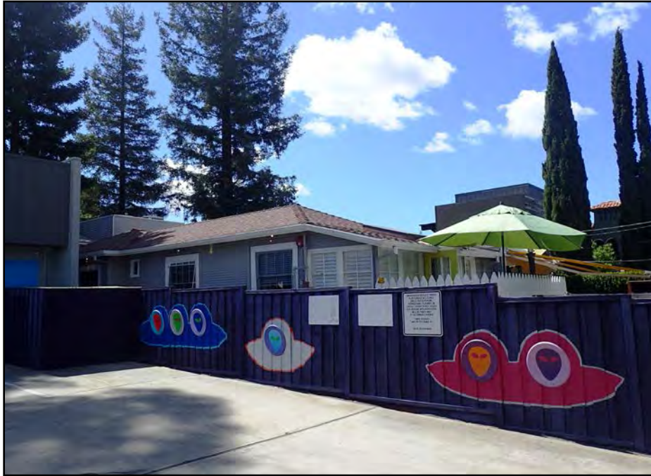
145 First Street, south and (partial) east façades. View to the northwest. LSA Photograph 5/13/17.
